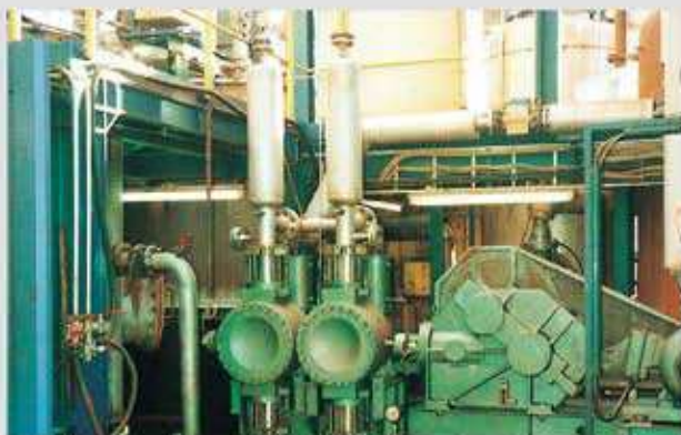
SG 130/135 - K 160 - 2 SM 350 HD Q = 3 - 20 m 3 /h p = 40 bar P = 55 kW Medium: Fe 2 O 3
