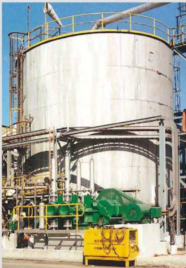
DG 180/200 - 2 K 180 - 4 SM 460 HD Q = 54 m 3 /h p = 64 bar P = 185 kW Medium: nickel ammonium sulphate sludge
