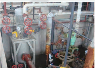
Replaced canned pump
